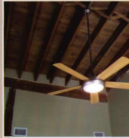
LARSON EXPOSED JOISTS & LIGHTING
